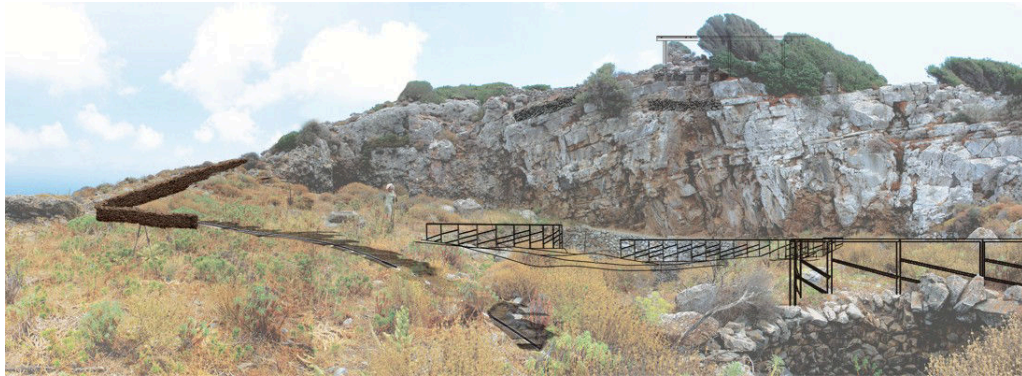
Figure 8: Dilakko cisterns area. The protection rails and the new drystone path.
