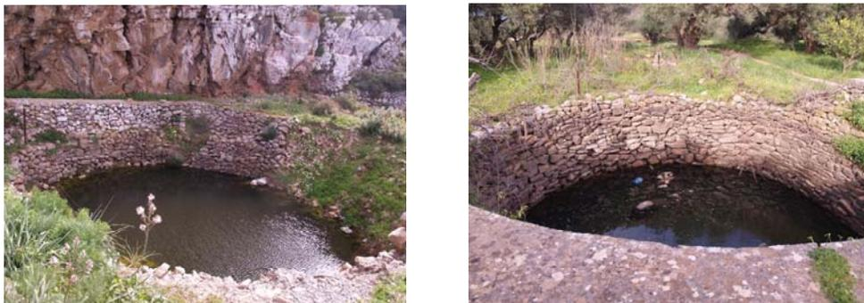
Figure 3: a) Large cistern in Dilakko, where a large section of the wall is collapsed and b) Circular cistern in Vrouchas, where section of wall and the concrete crown are collapsed.
